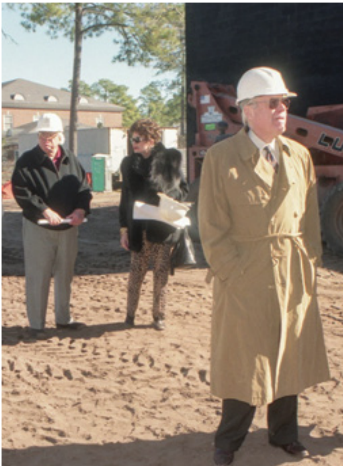
Thomas W. and Robin W. Edwards tour the Edwards Building construction site along with then-President Ronald Ingle.
